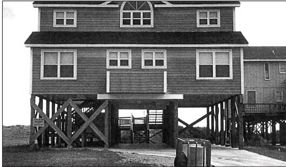
Figure 10-10. Diagonal bracing using dimensional lumber
